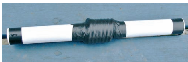
● Fig. 8: After the traps are held in place with tightly wrapped pvc insulating tape, they are ready to have the heavy duty waterproofing Denso tape wrapped around them.
